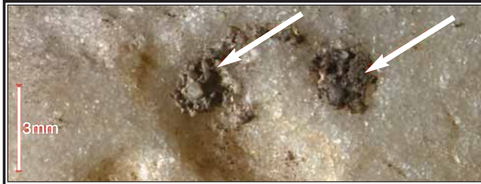
Figure 6: Small remnants of mortar inside a weathered cursive writing groove on the back side (white arrows).
